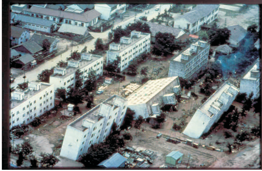
Figure 1.1: Group of apartment buildings in Niigata, Japan after a magnitude 6.5 earthquake rocked the town in 1964. The buildings failed due to loss of bearing capacity when the soil beneath liquefied (after Kramer [3]).
